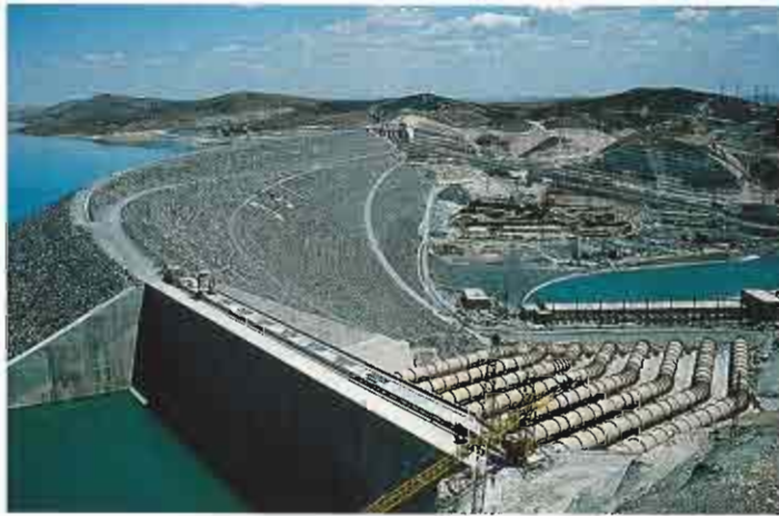
The hydropower plant at the Atatürk Dam has an installed capacity of 2,400 megawatts.
